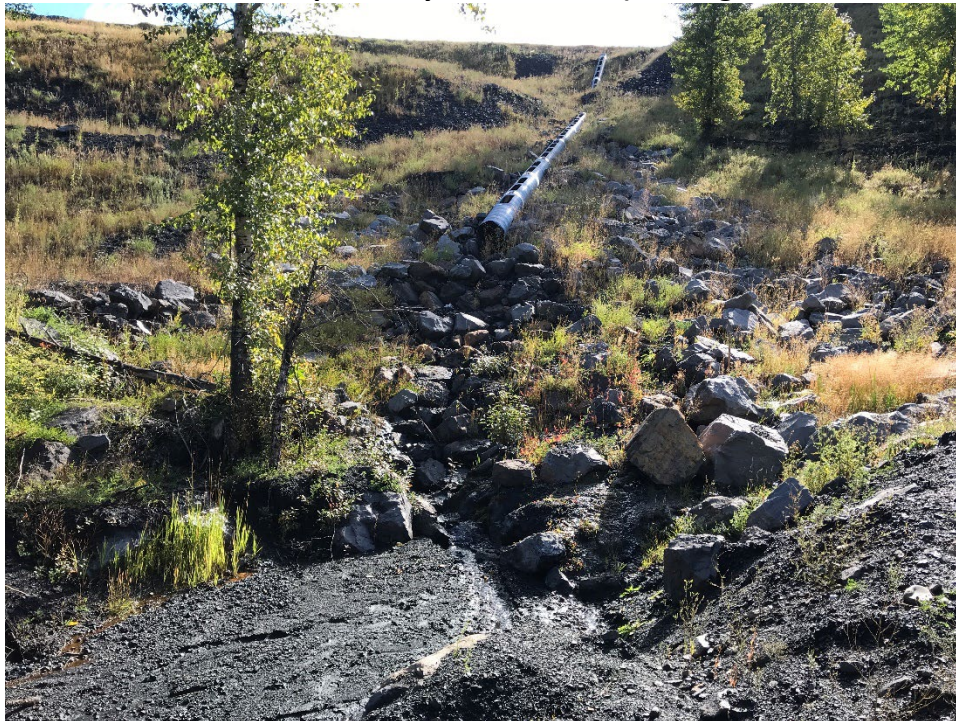
Photo I-4 CCR Dump Lindsay Drain outlet. (Looking east – Taken 20 September 2022)
