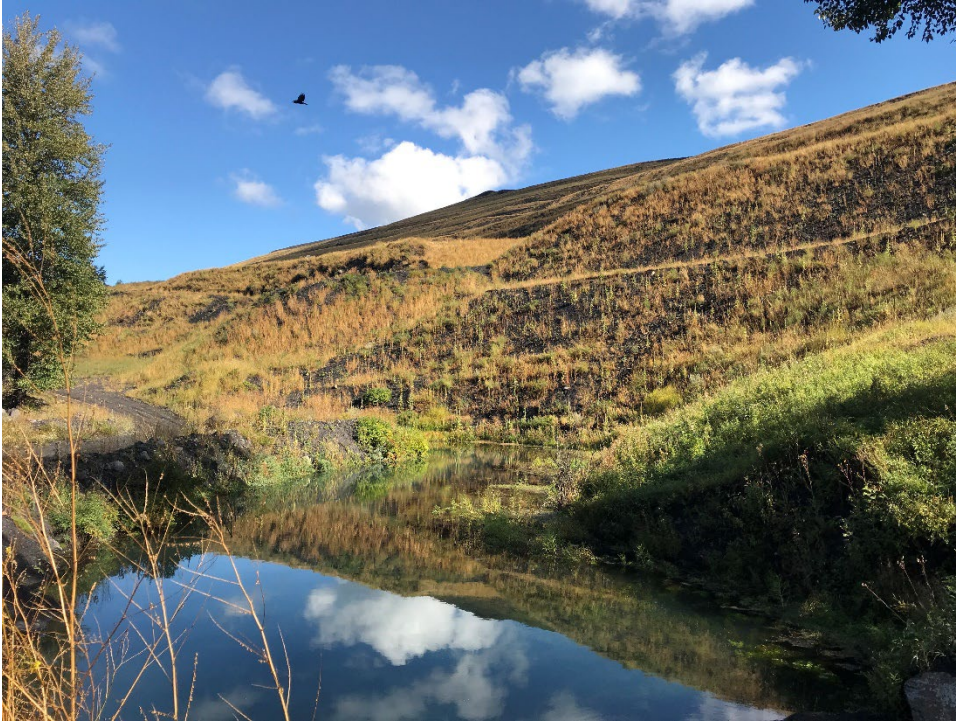
Photo I-3 CCR Dump toe sedimentation ponds. (Looking NE – Taken 20 September 2022)
