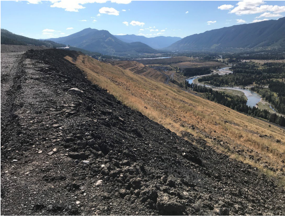
Photo I-9 CCR Dump crest and slope benches typical condition. (Looking south – Taken 20 September 2022)
