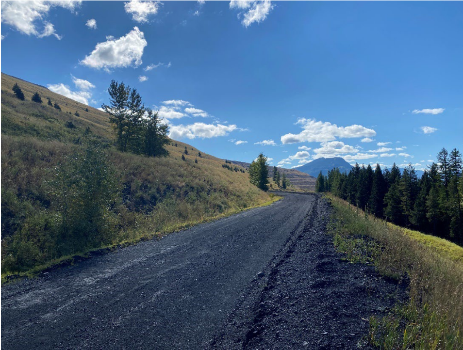
Photo I-7 CCR Dump slope benches typical condition. Seepage present in upstream ditch. (Looking south – Taken 20 September 2022)
