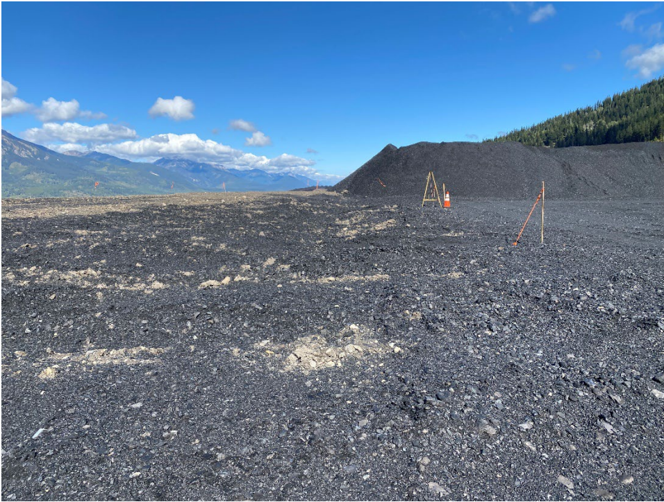
Photo I-15 CCR Dump surficial cracking behind crest, with monitoring instruments. (Looking north – Taken 20 September 2022)
