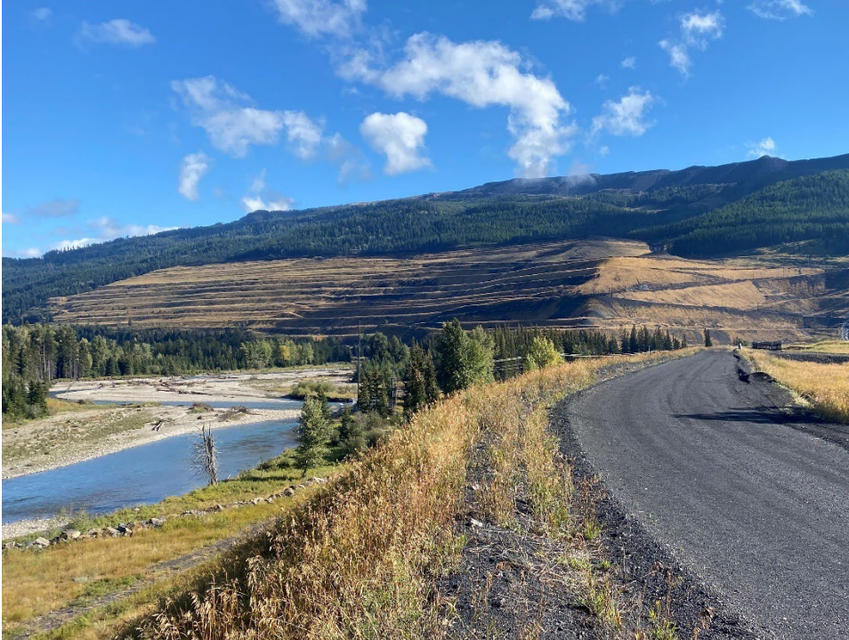
Photo I-1 CCR Dump overview. (Looking NE, from Lagoon C crest – Taken 20 September 2022)
