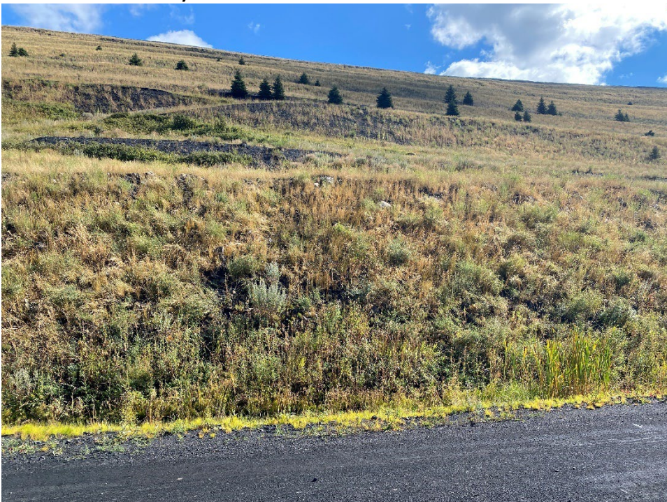
Photo I-8 CCR Dump slope benches typical condition. (Looking east – Taken 20 September 2022)
