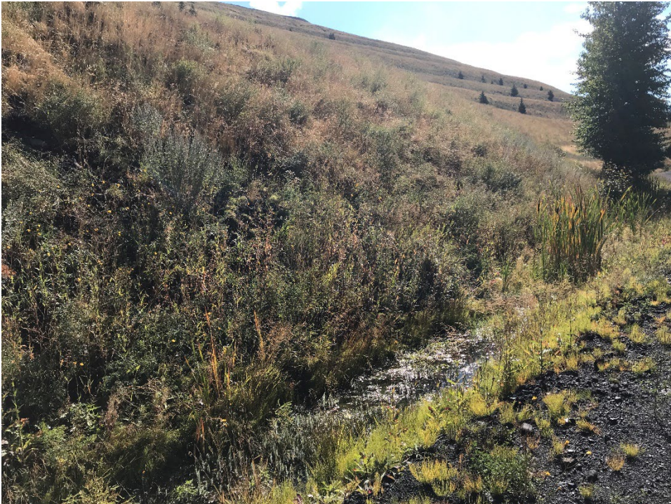
Photo I-6 CCR Dump seepage at bench ditches. (Looking SE – Taken 20 September 2022)
