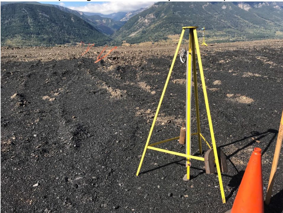
Photo I-16 CCR Dump crack meter instrument monitoring for surficial cracking behind crest. (Looking west – Taken 20 September 2022)
