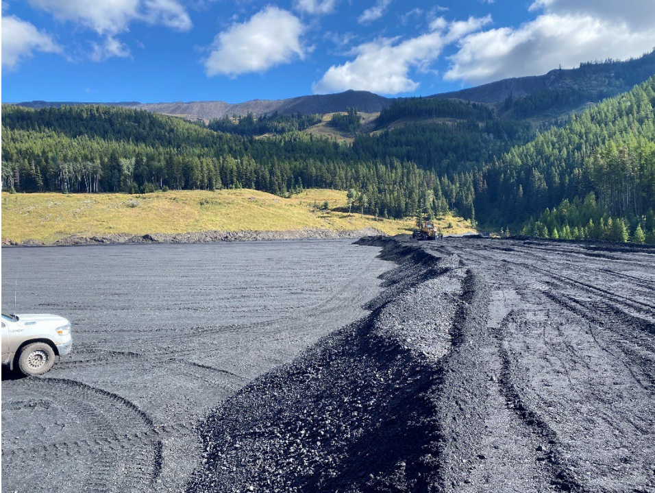
Photo I-11 CCR Dump crest pad material placement. (Looking east – Taken 20 September 2022)
